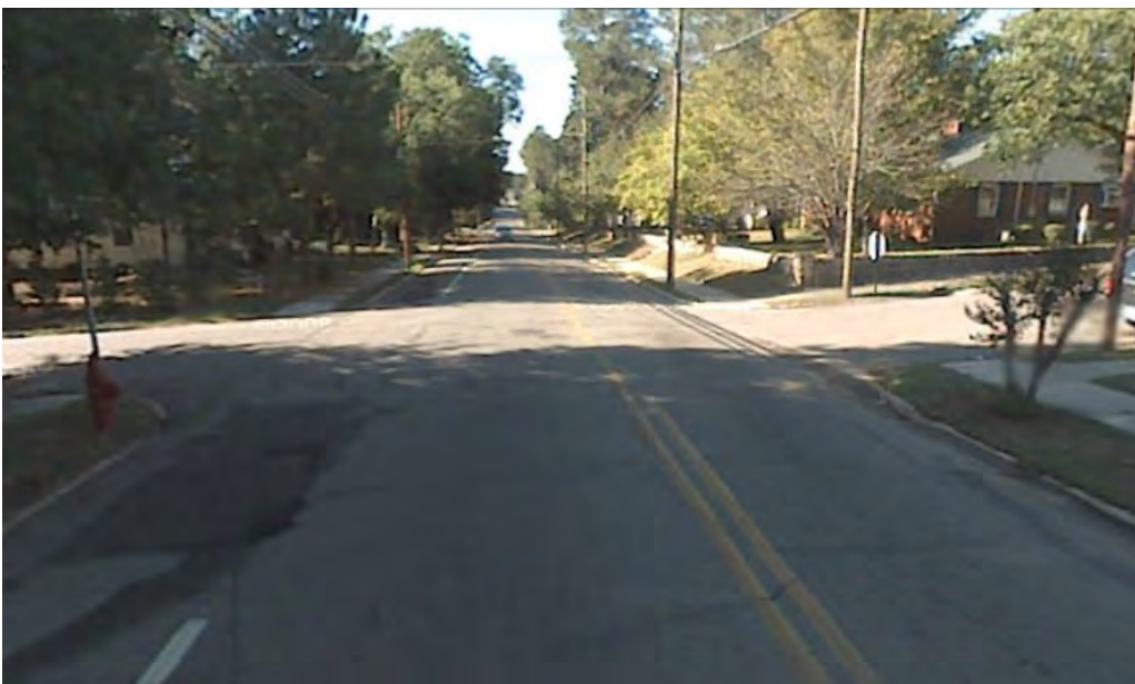
Left: Poplar Street, at Elm Street crossing. High-visibility marked crosswalk, a curb bulbout, and pedestrian crossing signage would be appropriate here.
